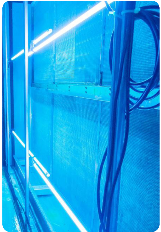
The RLM Xtreme fixtureless UV-C lamp system generates up to twice the ultraviolet irradiation levels as fixtured lamp systems.
