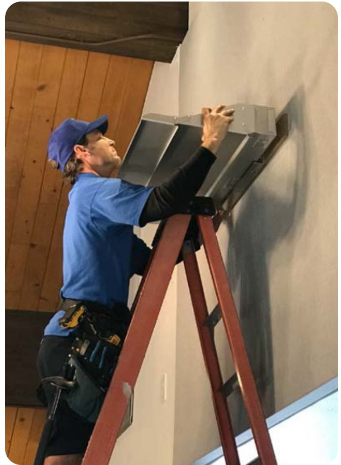
The UV disinfection fixtures are active when congregants are in the sanctuary and during choir practice.
