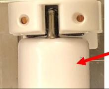
Insert the pins of the lamp straight down into the Tombstone on each end of the fixture (as shown)
