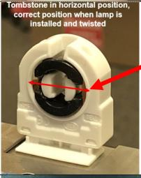
Holding the newly inserted lamp by both lamp end caps, rotate entire lamp a quarter (1/4) turn. The lamp pins will now be in a Horizontal position as shown in the picture to the left.
